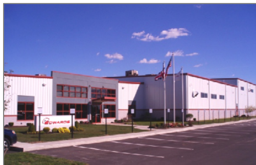
The Edwards Vacuum facility is located at Vantage International Point in Sanborn, New York.
