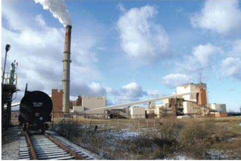
Riesling Power, LLC owns and operates the Somerset Power Plant on the southern shore of Lake Ontario. It produces electricity at its 675 megawatt coal-fired generating plant. Its 1,200 acre site receives bituminous coal by way of rail lines owned by the Somerset Railroad Corporation.
